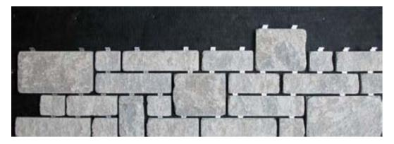
Figure 2. "Shouldice Fusion Stone" installed for the Grouted Joint Design Just Before Grouted
